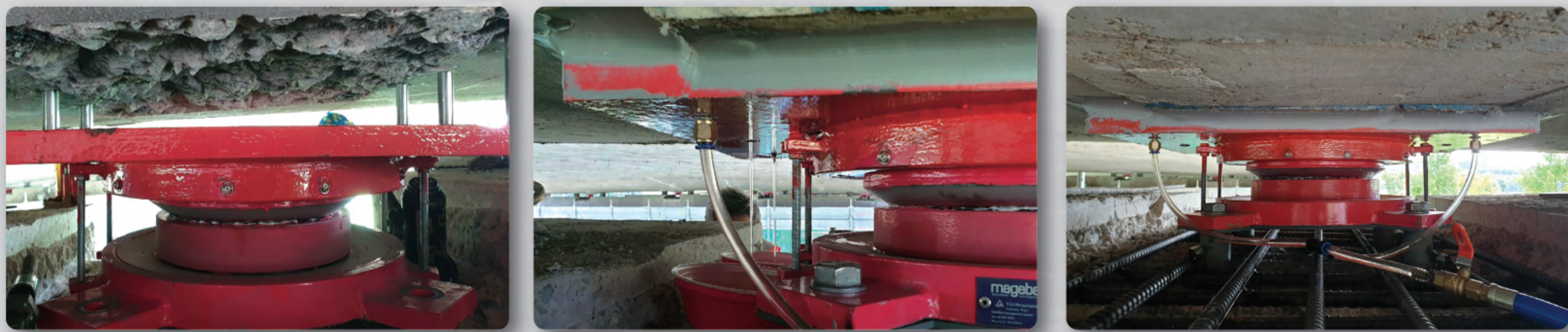
Epoxy Perfect Filling Method for the Bridge Bearing Replacement
